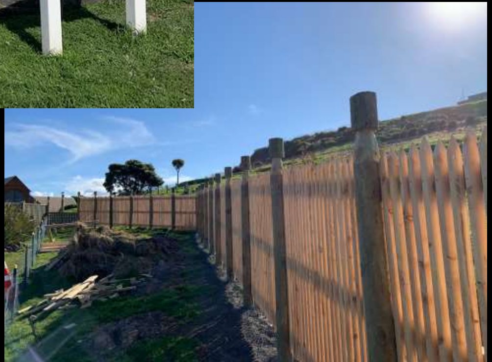
Palisade security fence
